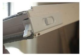
And here's a new one installed. It just pressed into place and is located by the lugs on the body of the latch.
