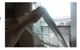
Grip the bottom part of the latch with the pliers and give a good hard tug on it. It will slide out and you can see all of the latch to compare it to pictures of replacement ones.
