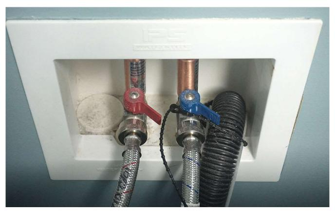
You can leave the large plastic drain hose connected if you aren't going to stretch it out too much, but if you want to take it out of the wall recess you can unhook the reusable beaded plastic safety cord that keeps it in place. Just be sure not to lay the drain hose flat – it probably has some water in it.
