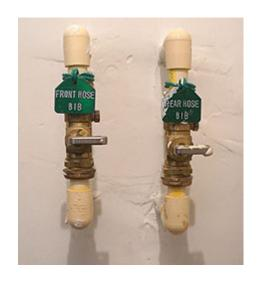
**Get an old towel or rag and a catch basin** and hold the basin below one valve. Using a pair of pliers, *gently* grip the little brass vent plug (red arrow in the picture) and unscrew it just until it moves. Using your fingers, unscrew it further *very slowly*.
